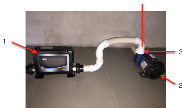
1. Elbox 2. Pump 3. Snabbkoppling
